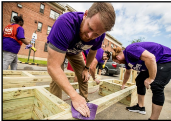
LS Morgan Cox KaBoom! Playground Build
